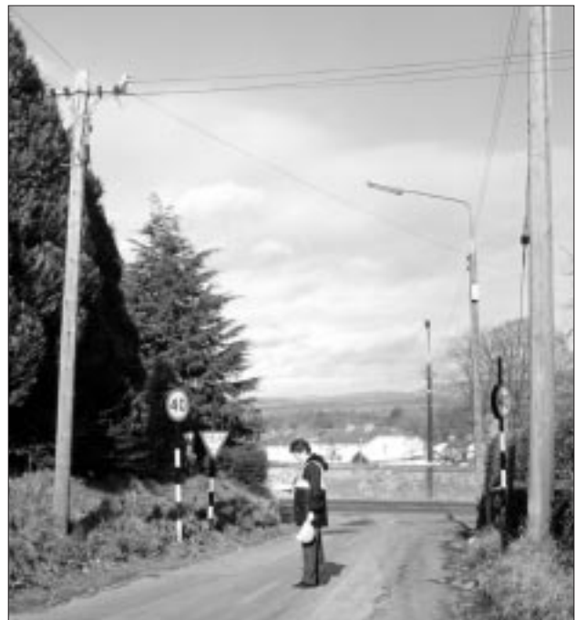
The CHM2000 being used to measure the height of the overhead cable
