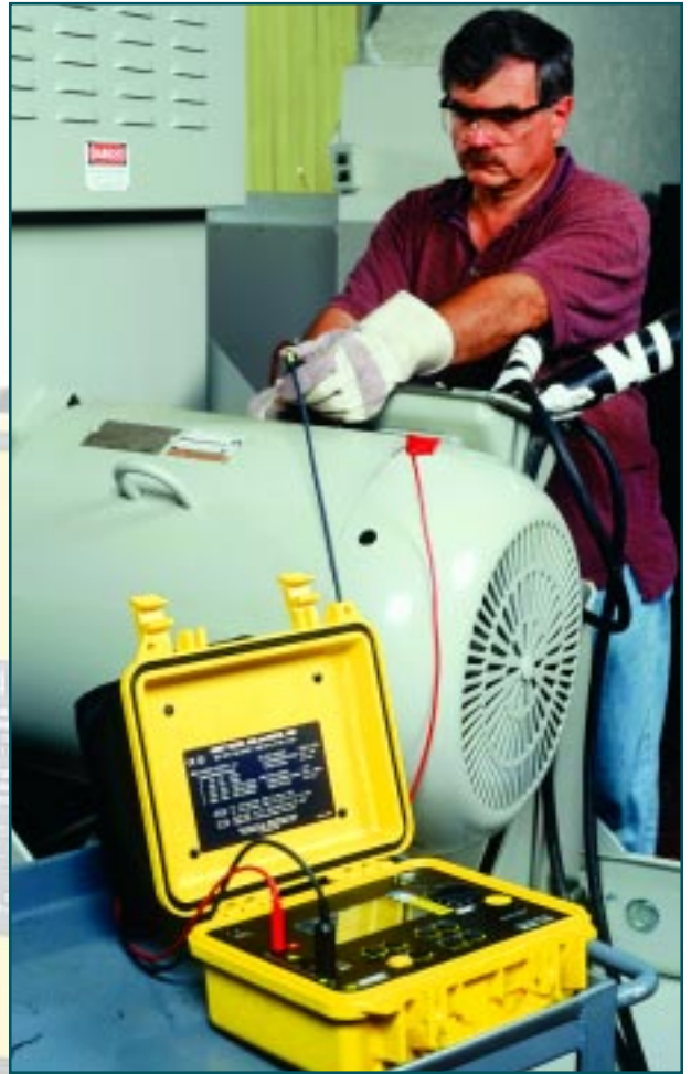
Model 1060 checking insulation resistance between windings on a 3 phase motor.
