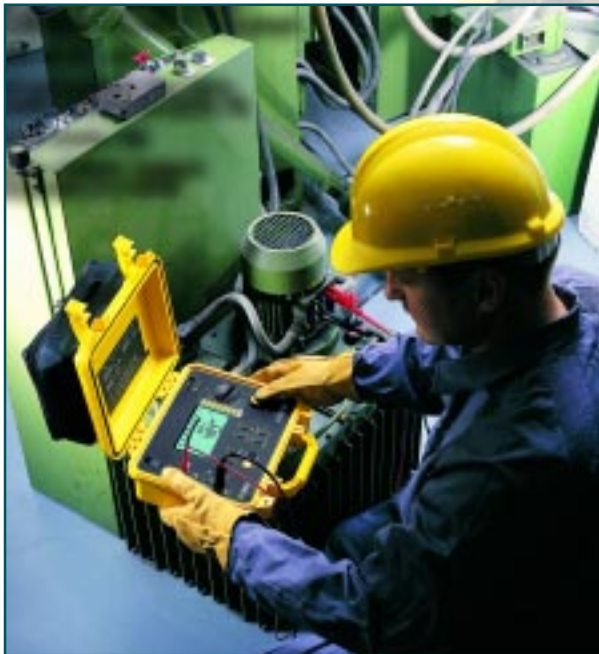
Model 1060 performing insulation test on contacts of a generator.
