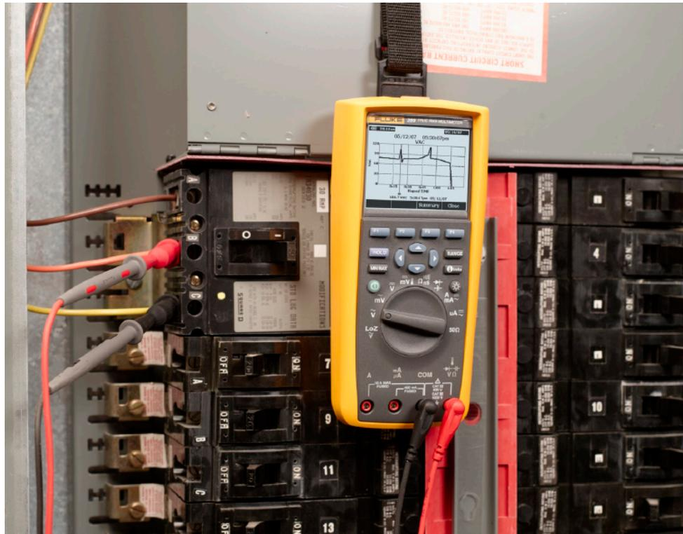
occurred, based on the start of the monitoring process. The actual start time for the Min Max session is also displayed so it is relatively easy to determine exactly when the signal changes have occurred.
