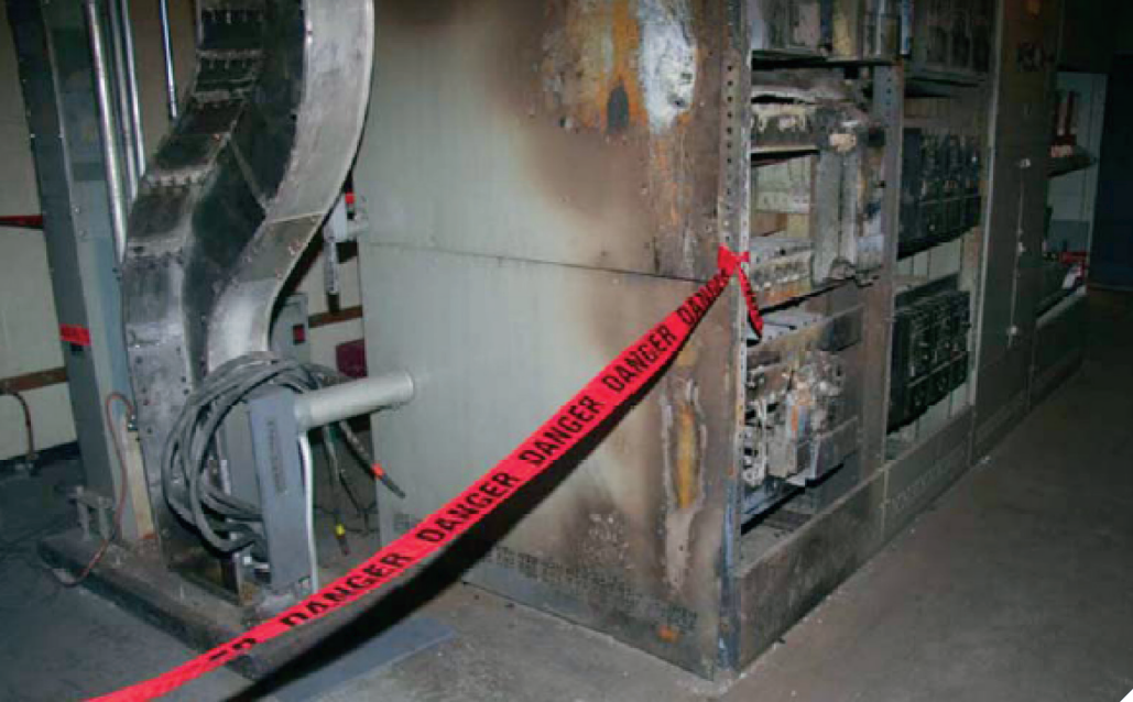
Figure 2. Switchgear fire that resulted in $2.7 million in damage. This facility declined an IR survey offer by a CNA thermographer just months before the fire happened.
